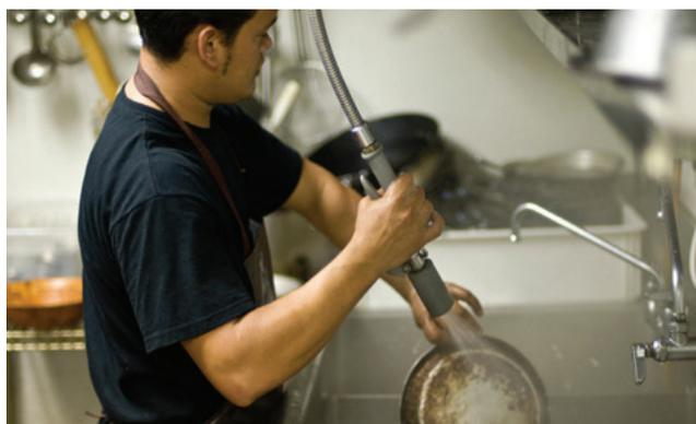
water to rinse dishes, installing a WaterSense labeled pre-rinse spray valve can reduce a commercial kitchen's annual natural gas use by more than 6,400 cubic feet per year. That's enough energy to run its convection oven 12 hours a day for three weeks.
