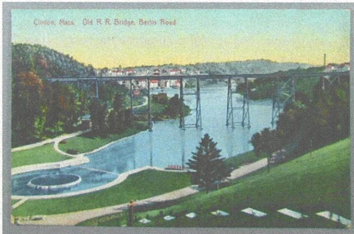
Old Railroad Bridge, Berlin Road, Clinton MA
